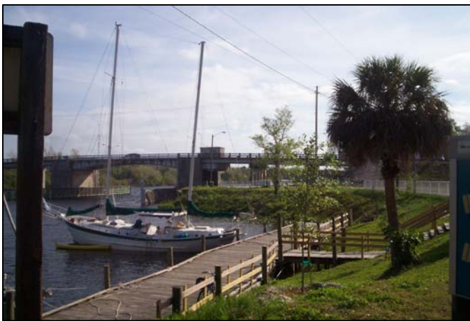
View of Existing Wharf
